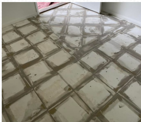
Filling Grout Lines Over Tiles
